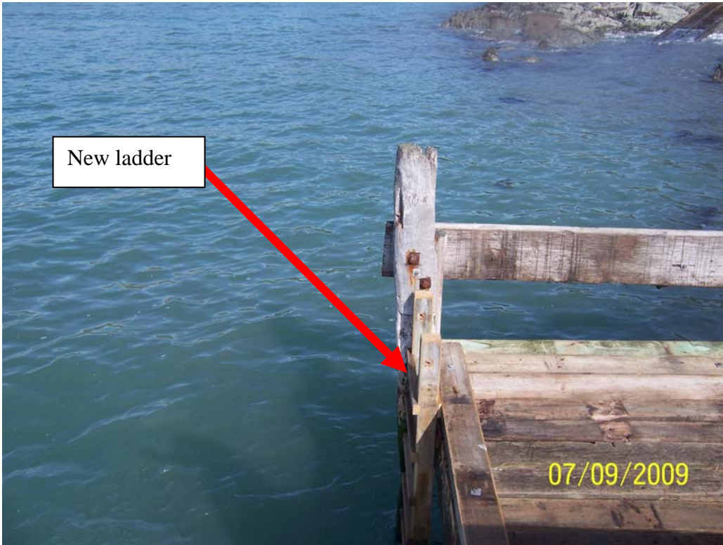
The new ladder giving access to sea level
