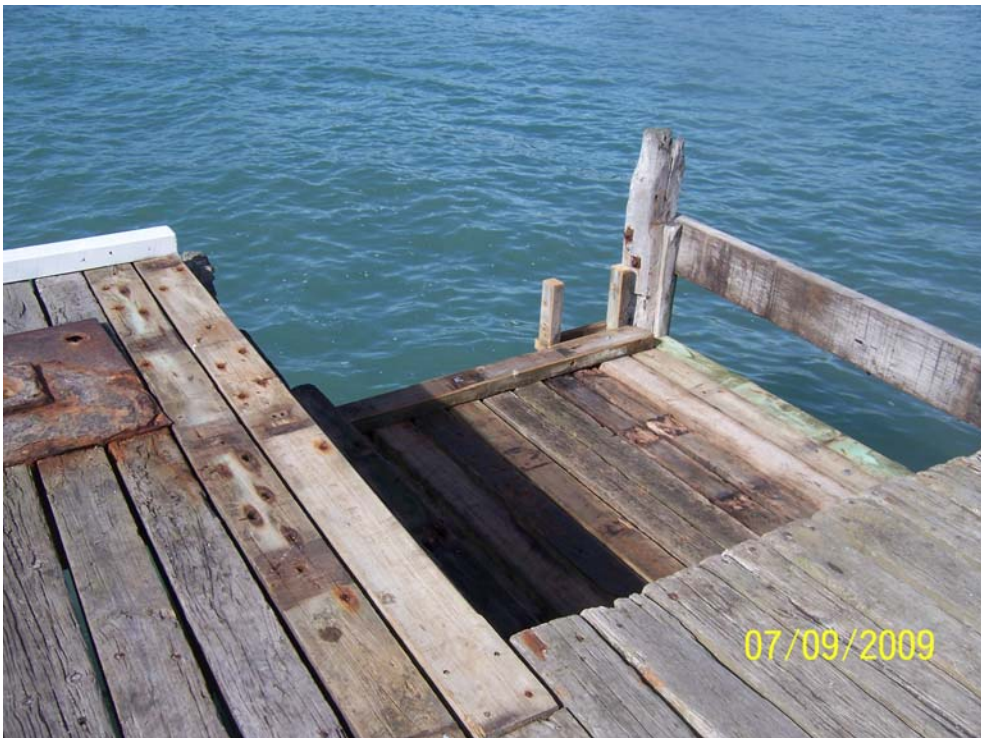
The platform has now been completely rebuilt
