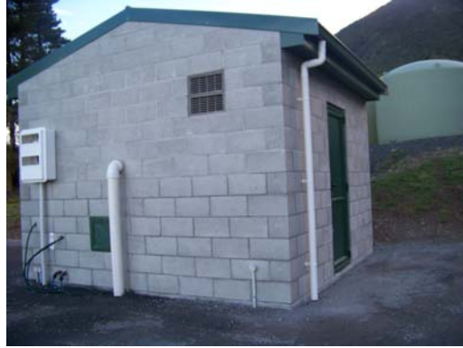
Figure 2: Newly build treatment Shed - Kincaid Supply
