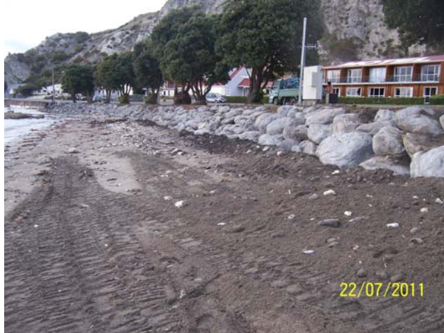
Figure 6: Rock Wall to reduce the impact of erosion along Esplanade
