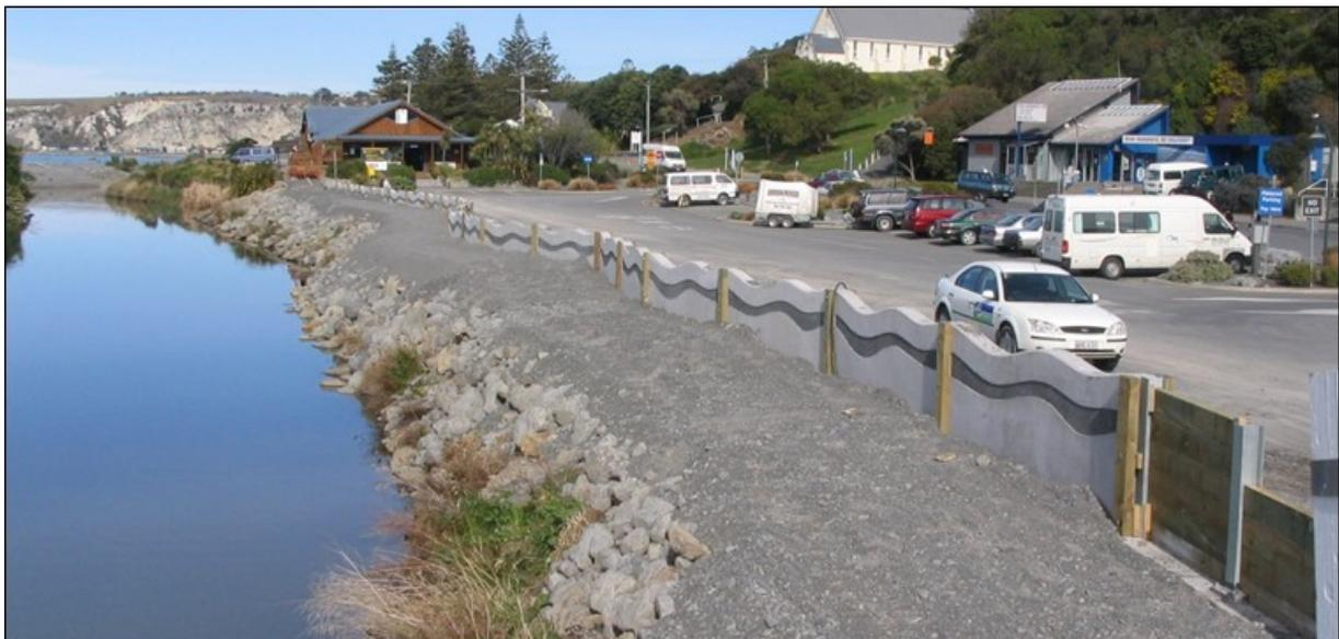
**Figure 2-8: Lyell Creek flood protection wall**
