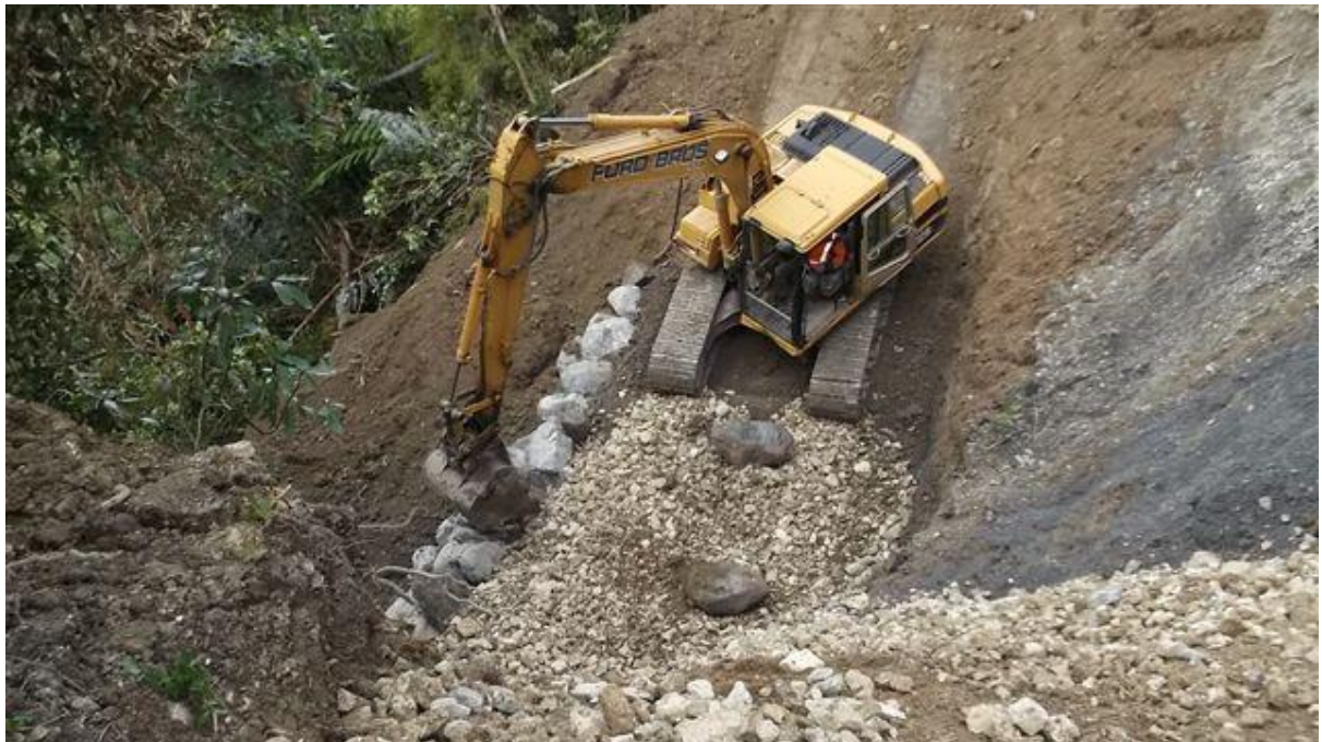
Figure 1. Repairs to slip on Blue Duck Valley Road
