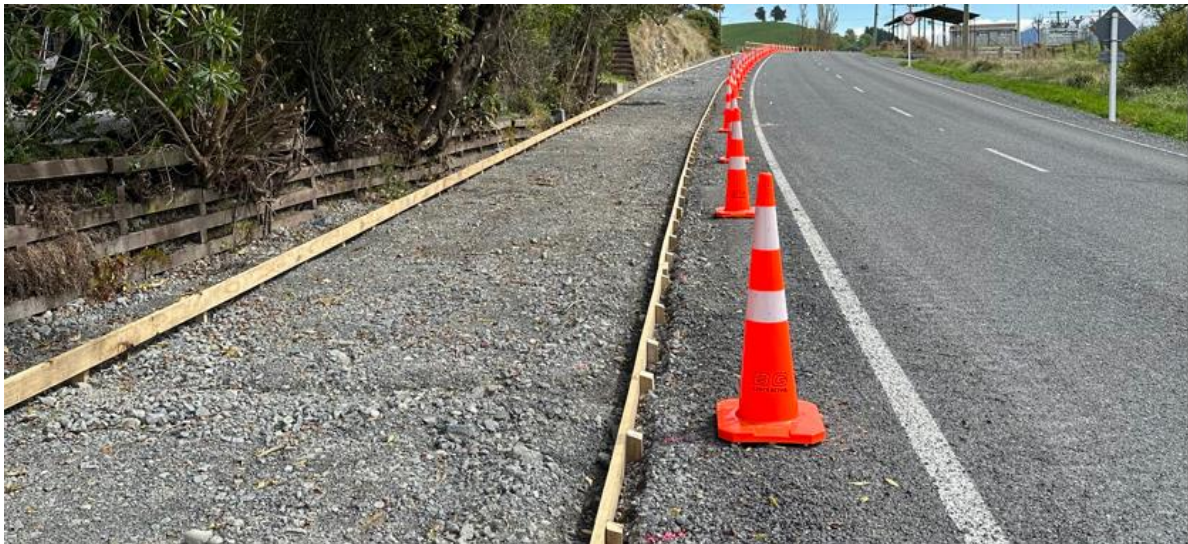
Photo 4: Shared user path (SUP) preparation works in Ludstone Road.
