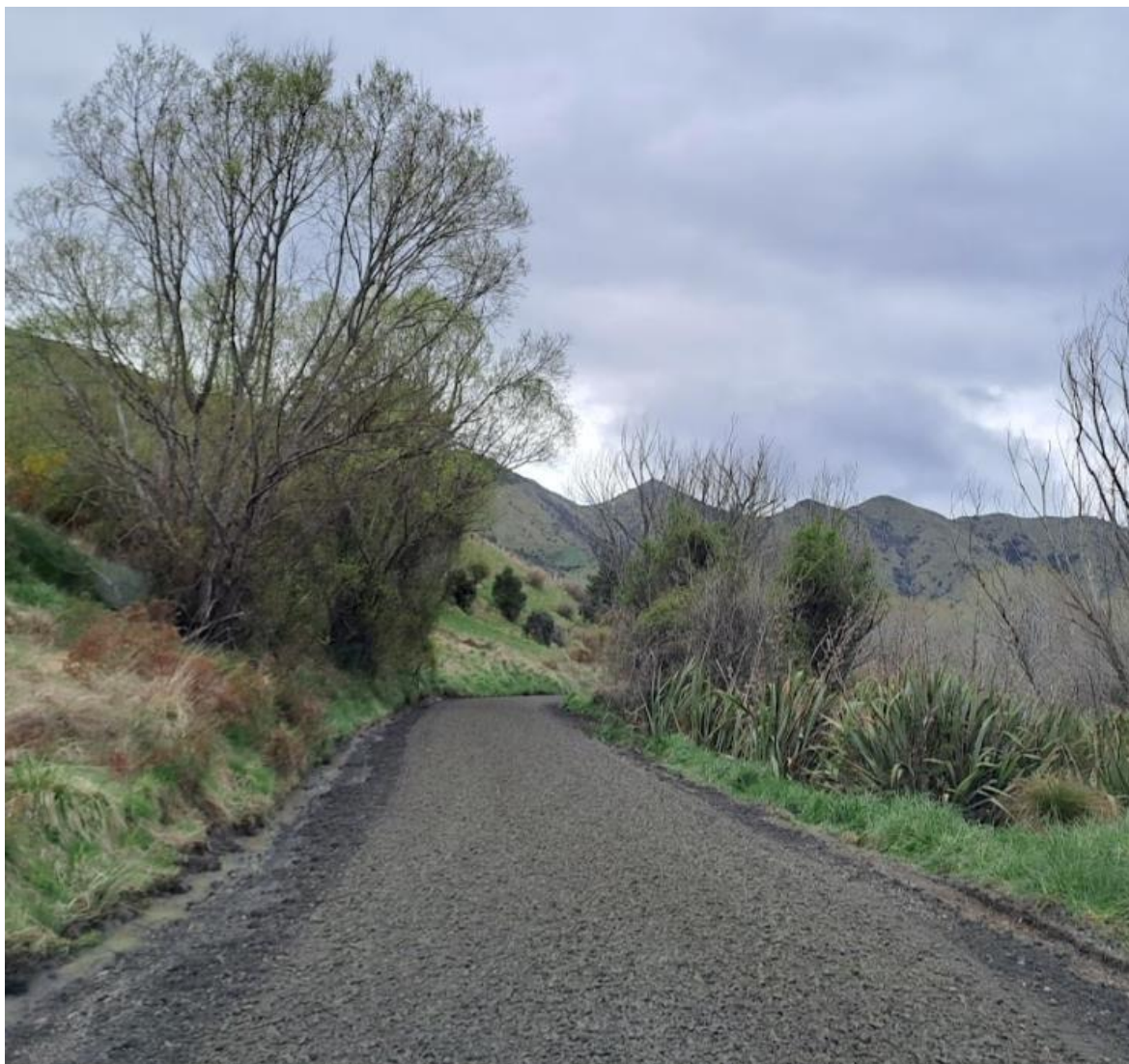
Photo 1: Metalling Blunts Road
