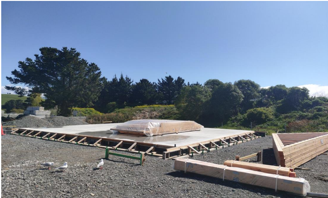
Photo 8: Re-Use Shop Construction
