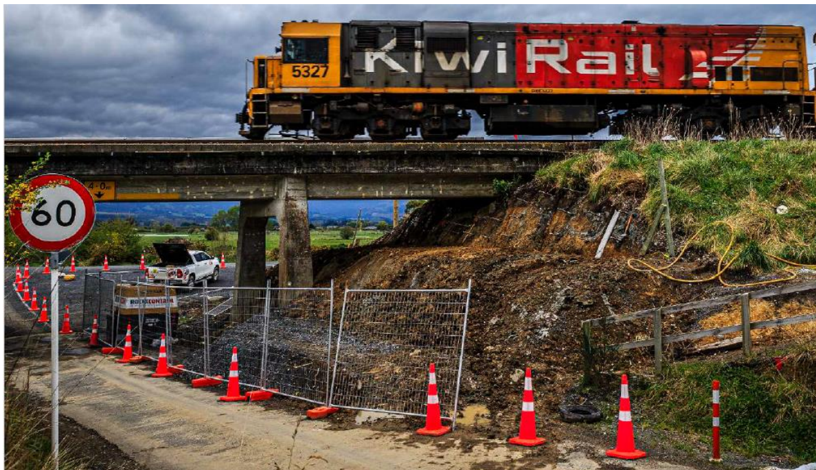
Photo 5: Soil nail installation under the KiwiRail Bridge 104
