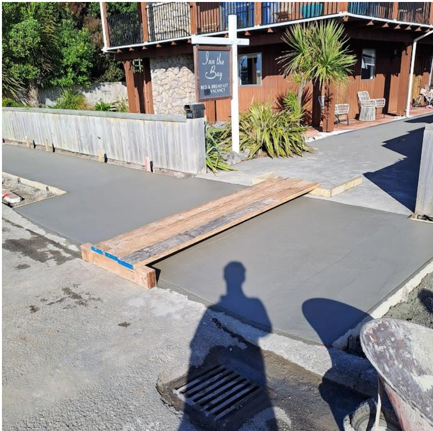
Photo 2: New footpath with pedestrian bridge at Esplanade.
