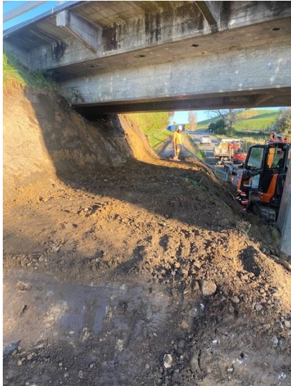
Photo 3: Bench excavation under KR104
