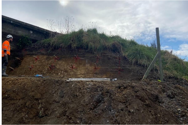
Photo 4: Soil Nail locations marked out on the embankment for KR104
