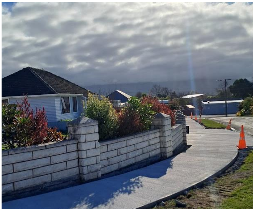
New footpath on Kiwi St
