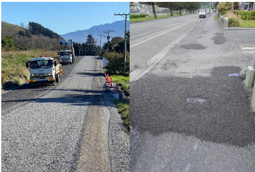
Left Sealing at Ludstone Road, Right chip seal footpath repairs
