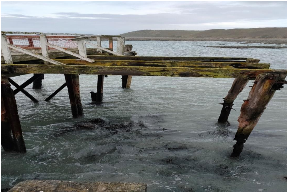
Old beams that need to be removed
