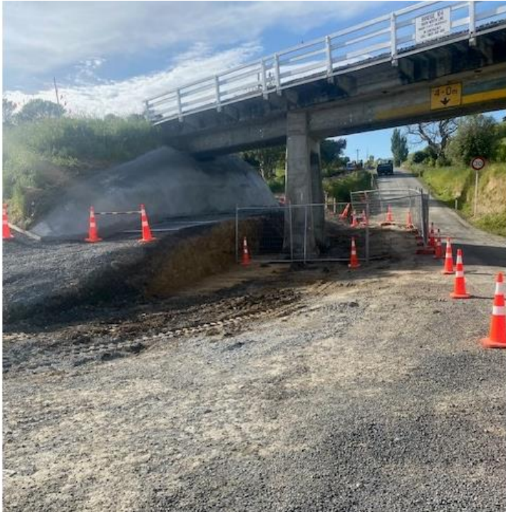
Photo 1: Rail bridge embankment excavation completed ready for gabion wall installation.
