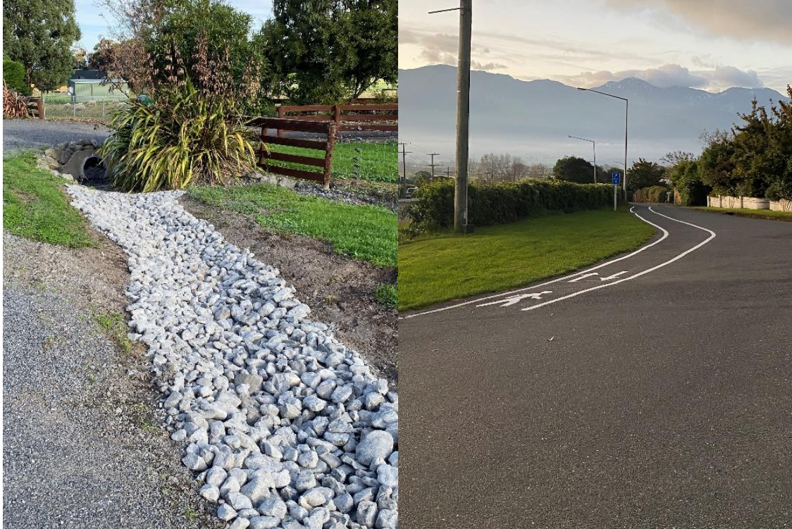
Left Gabion stone swale at Bay paddock Road Right new linemarking Adelphi Tce
