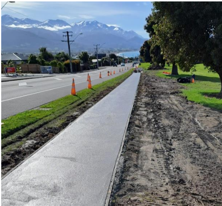
Photo 2: New footpath on Churchill Street near completion
