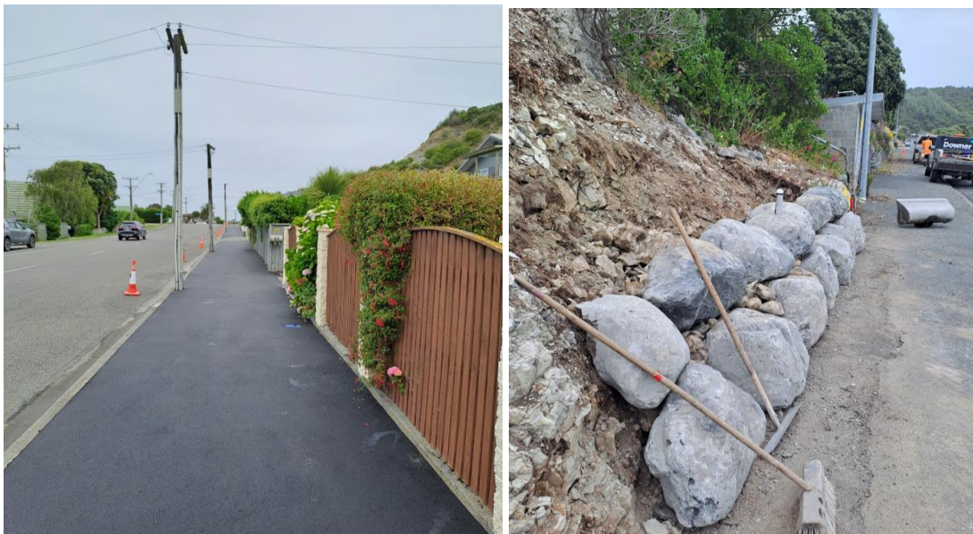
New surfacing at Avoca left and new rock retaining wall right
