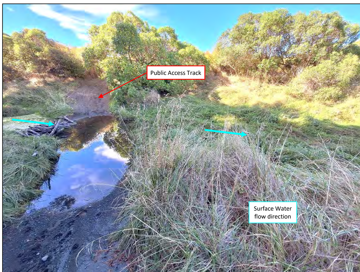
Figure 34: Stormwater Flowing to Sea, and Crossing Access Track
