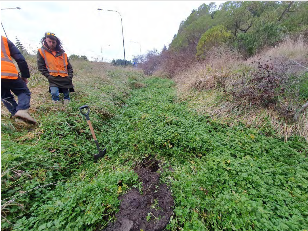
P10: View of open drain south-west of twin 900 outlet. A hand dug test pit was also excavated here, which found topsoil.
