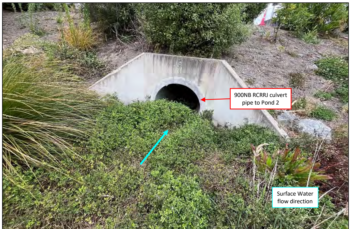
Figure 28: Upstream Catchment Flow Through 450NB then 900NB RCRRJ Culvert Pipes to Pond 2
