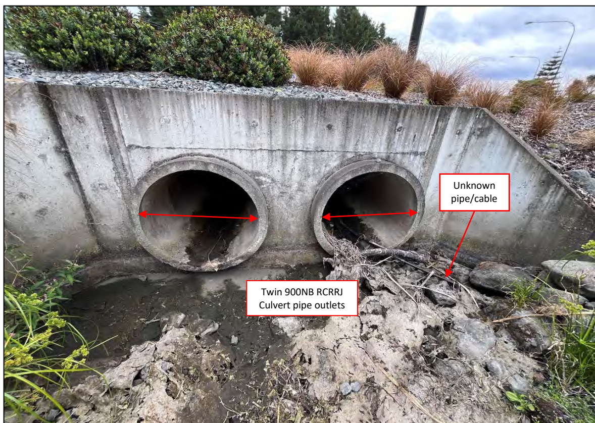
Figure 20: Pond 1 twin 900NB RCRRJ culvert pipe outlets crossing SH1 (closer look)
