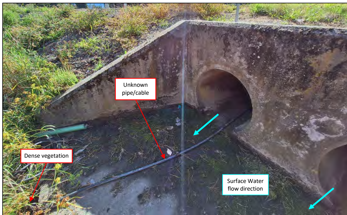
Figure 21: Twin 900NB RCRRJ culvert pipe south of SH1
