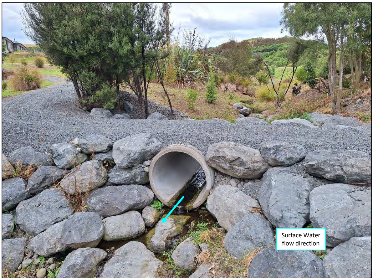
Figure 9: Pond 6 900NB RCRRJ Inlet from Pond 7
