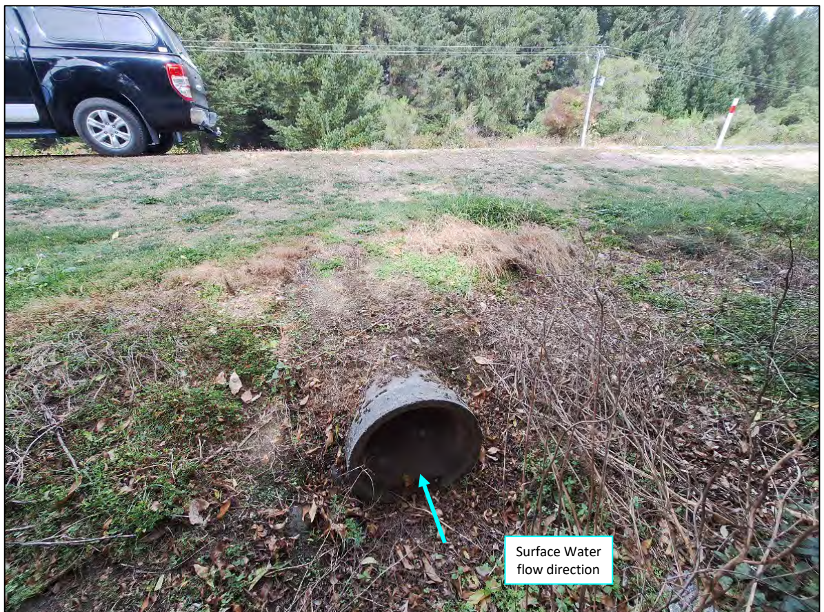
Figure 6: 450NB RCRRJ Culvert Inlet Discharging from the Golf Course (Crossing SH1)
