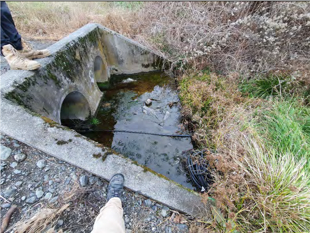
P12: View of twin 900 outlets at eastern end of open drain.
