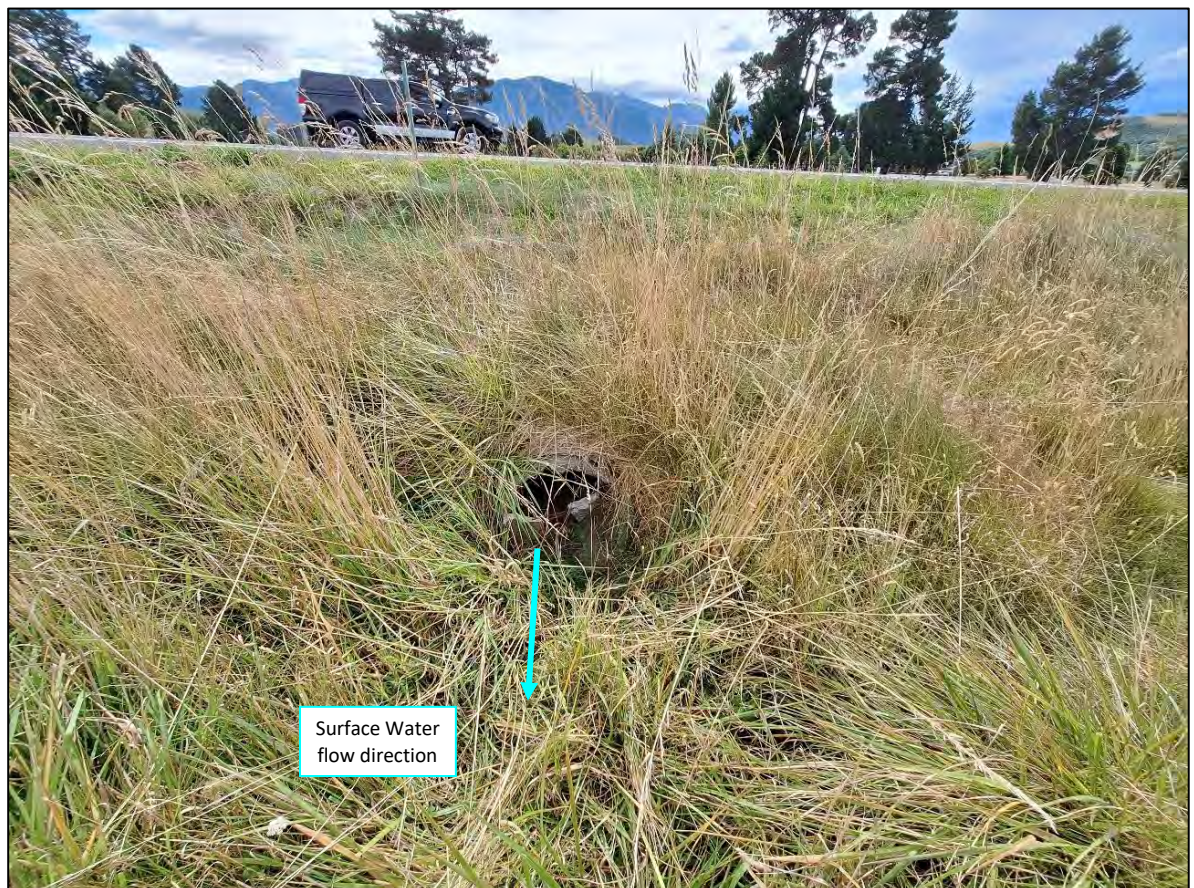
Figure 4: 450NB RCRRJ Culvert Outlet Discharging from the Golf Course (Crossing SH1)
