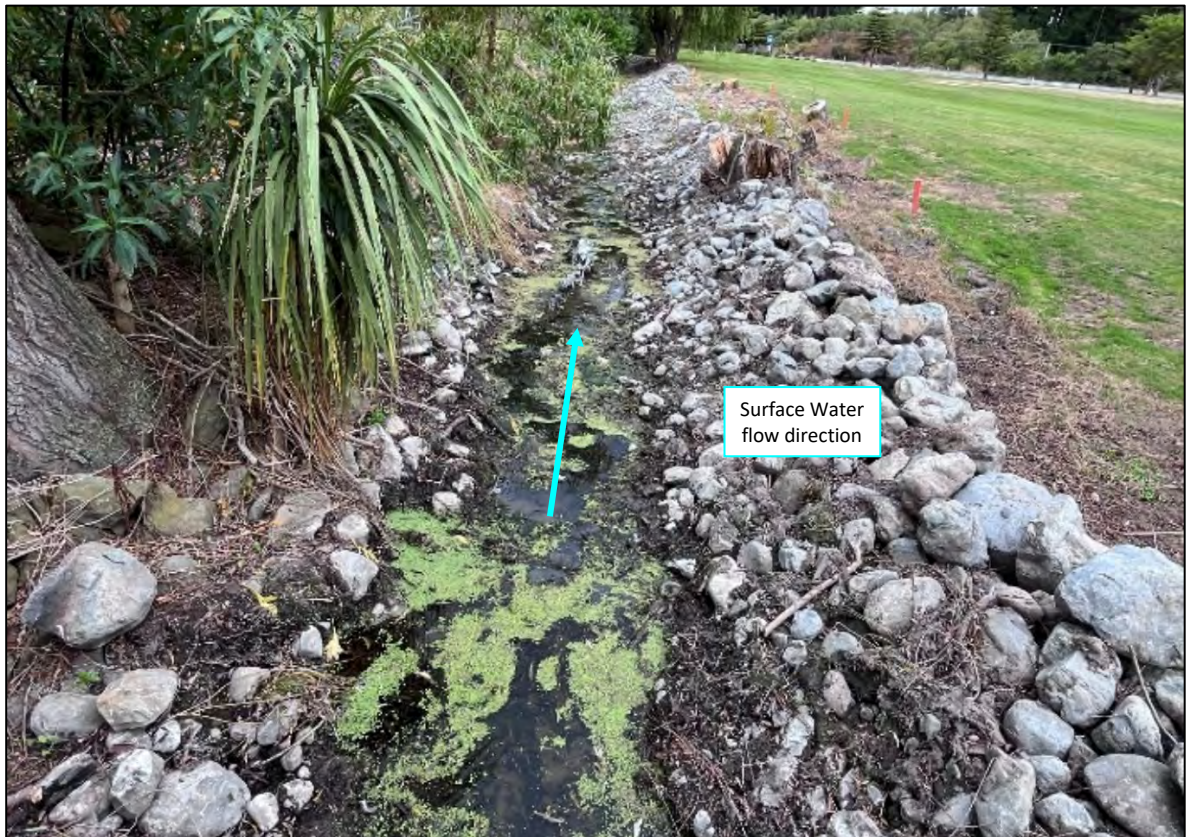
Figure 14: Open Channel from Pond 4 to Pond 3
