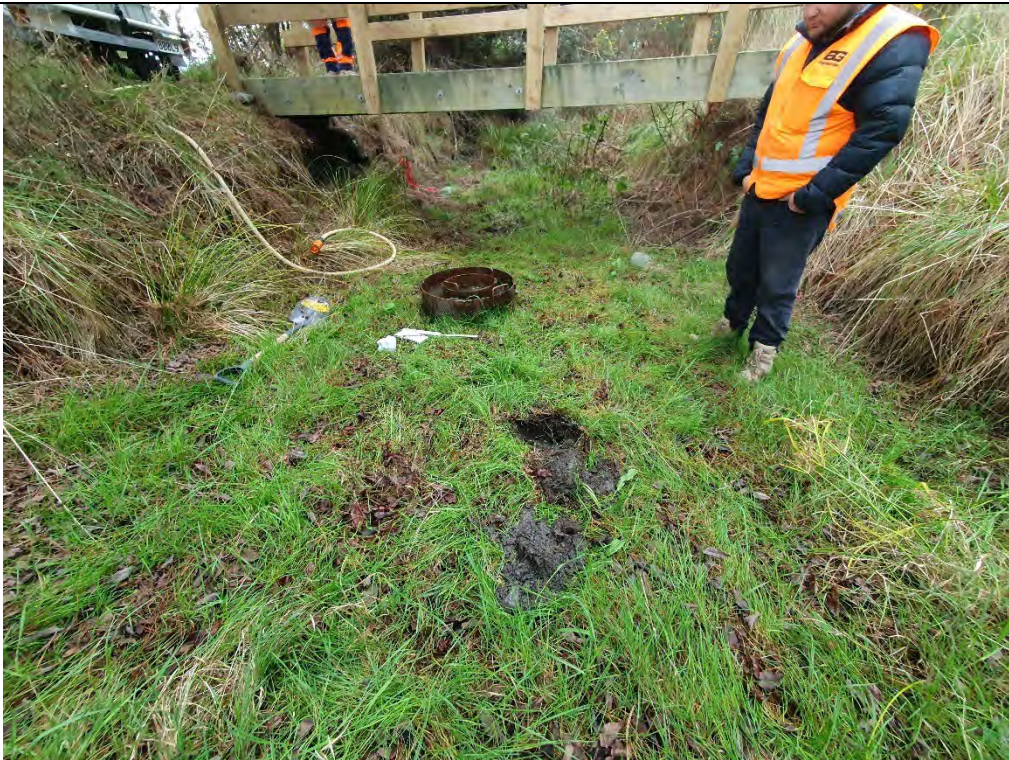
P6: Double-ring test DR4 and hand dug test pit located in base of open drain.
