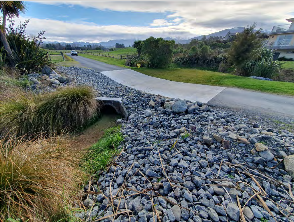
P14: View of weir located south of 21 Greenburn Way.
