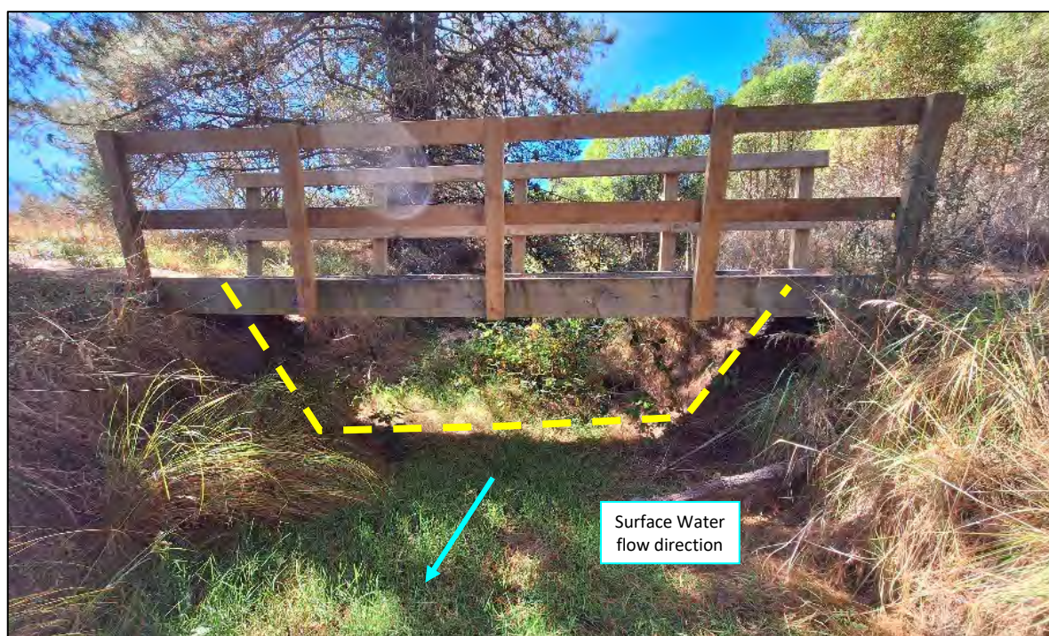
Figure 23: Bridge Crossing Flow Path/Channel from Twin 900NB and 450NB RCRRJ Culvert Pipes
