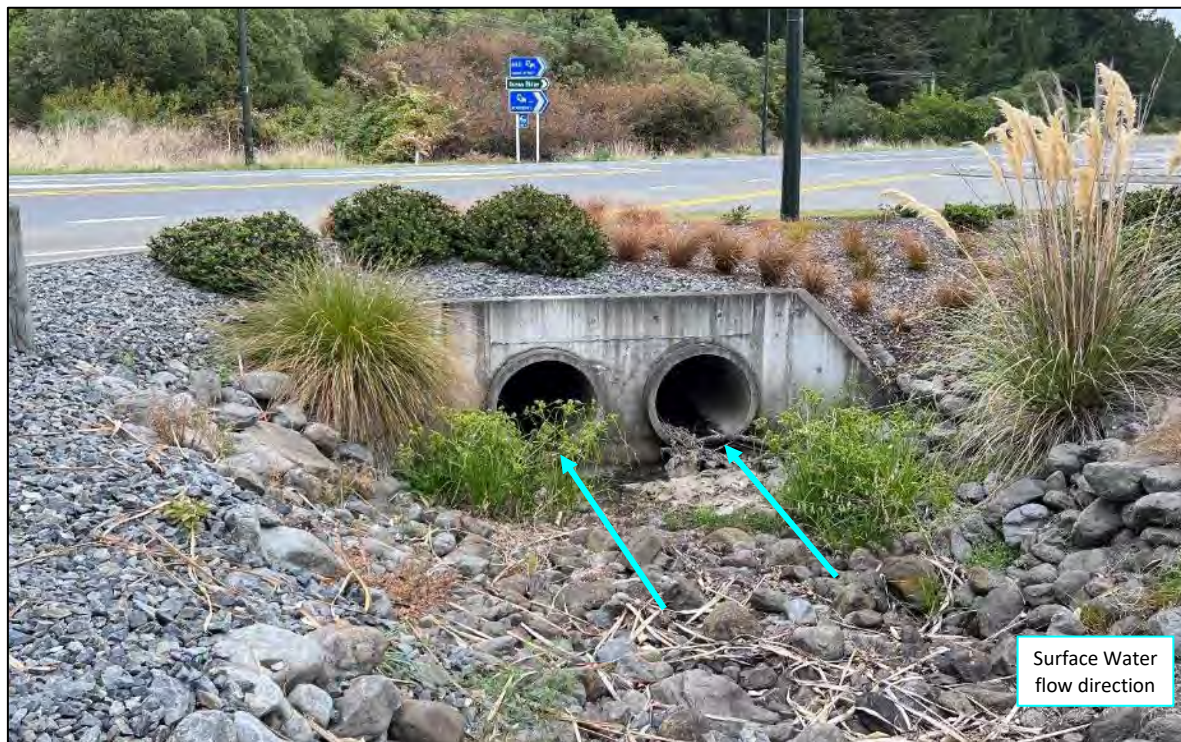
Figure 19: Pond 1 Outlet - Twin 900NB RCRRJ Culvert Pipes Crossing SH1
