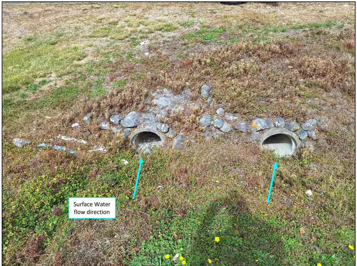
Figure 5: Twin 450NB RCRRJ Culvert Inlets Discharging from the Golf Course (Crossing SH1)
