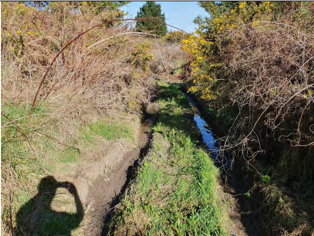
P8: View of open drain south-west of DR3. This section of open drain is not as well formed and has been used as a four wheel drive track, note the standing water in ruts. This section terminates at walking track that runs along the tops of the sand dunes to the south, and does not appear to outlet to the ocean.
