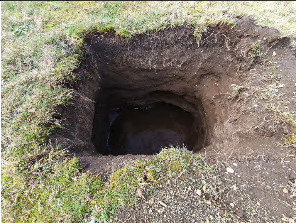
P1: TP1 after completion of infiltration test.
