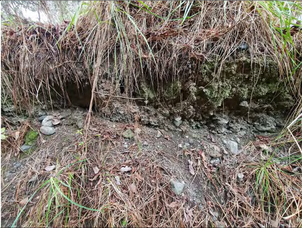
P7: View of side wall of open drain showing sandy silty gravels.
