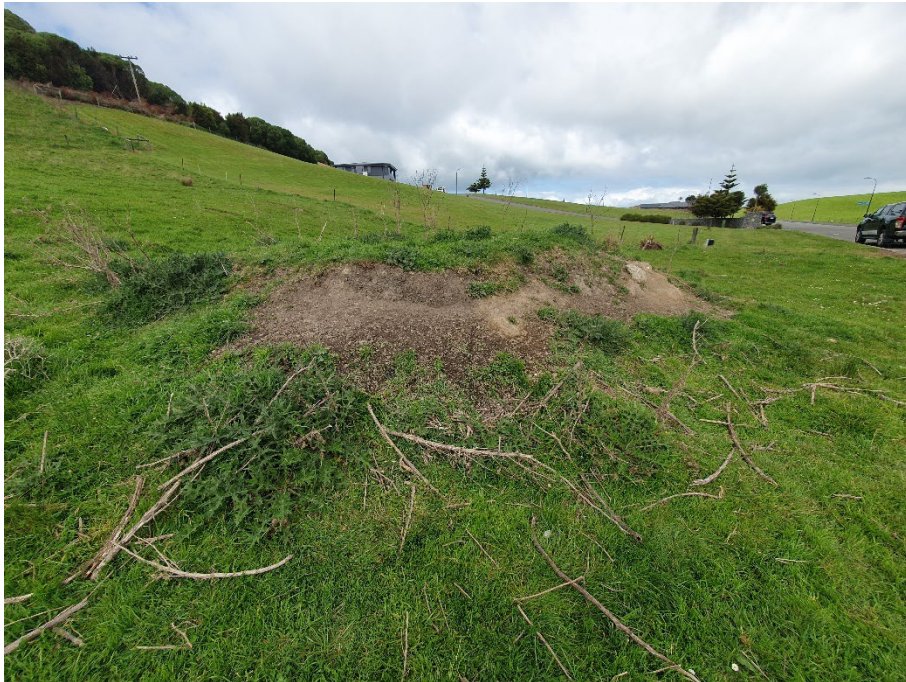
P26: Small sandy clayey silt stockpile located near south-western end of Area G. This stockpile is inferred to comprises excess soils from bulk earthworks or building construction in earlier stages of Ocean Ridge.
