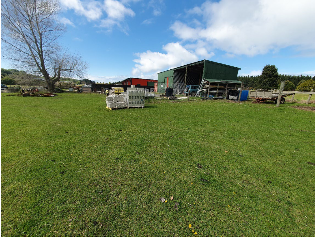
P7: Implement shed, circa 2012, located along the southern boundary of Area F. Various building materials, generally comprising concrete blocks, reinforcing steel and timber are being stored either on pallets or raised above ground.
