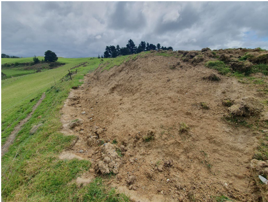
P17: Expsoed stockpiled sandy clayey silts (circa 2012).
