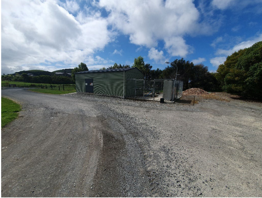
P15: Municipal water treatment facility, located to the east of the farm yard area. Signage indicates that Sodium Hypochlorite is used in the facility.
