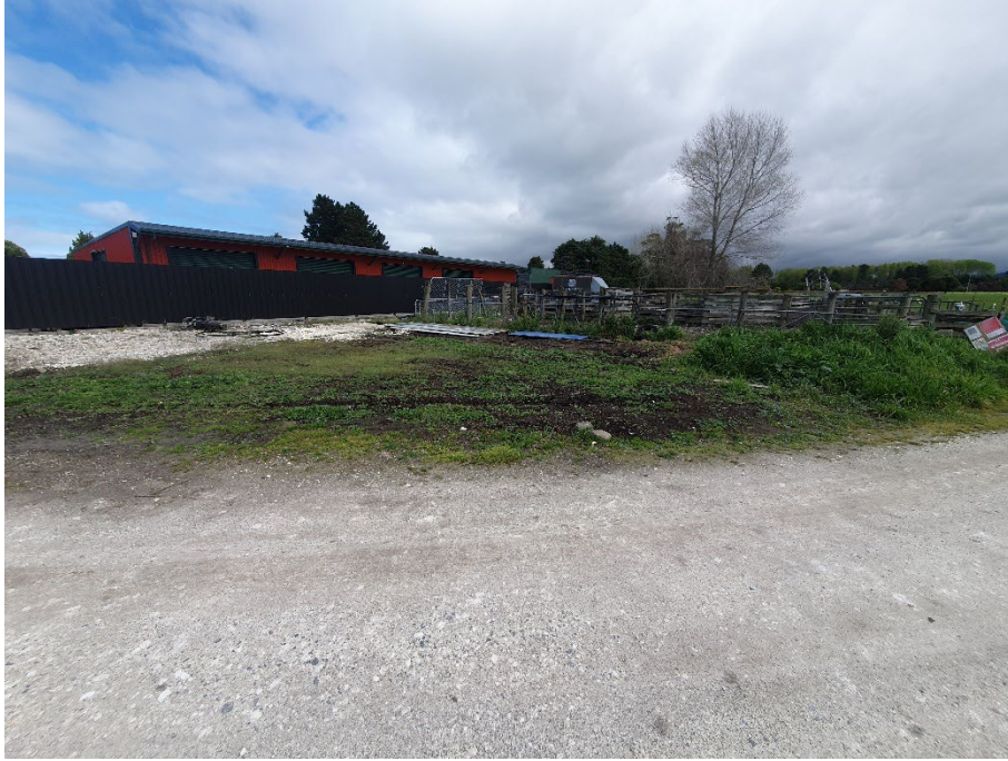
P13: View of recently constructed workshop building to the south of the stockyards.
