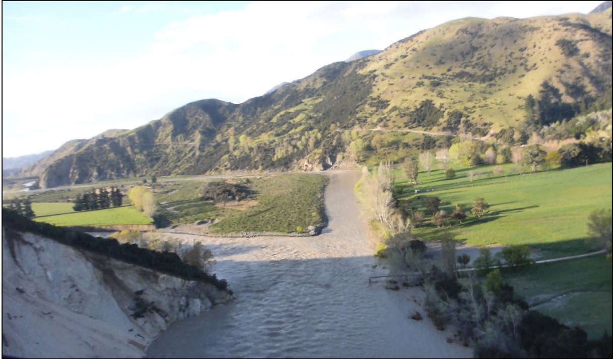
Figure 2-12: 27 September 2017 - Looking downstream at the destroyed Clarence Valley Road Bridge and new main Waiau Toa/Clarence River channel along the fault (left channel)
