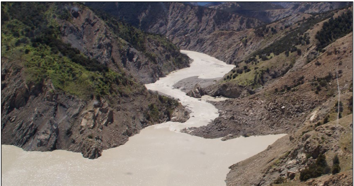
Figure 2-4: 15 November 2016 at 12:15pm - Looking downstream at the Waiau Toa/Clarence River landslide dam after it breached
