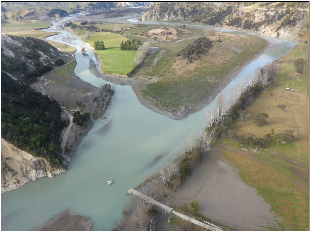
Figure 2-11: 18 July 2017 - Looking downstream from near the Clarence Valley Road Bridge to the new Waiau Toa/Clarence River channel running along the fault through farmland
