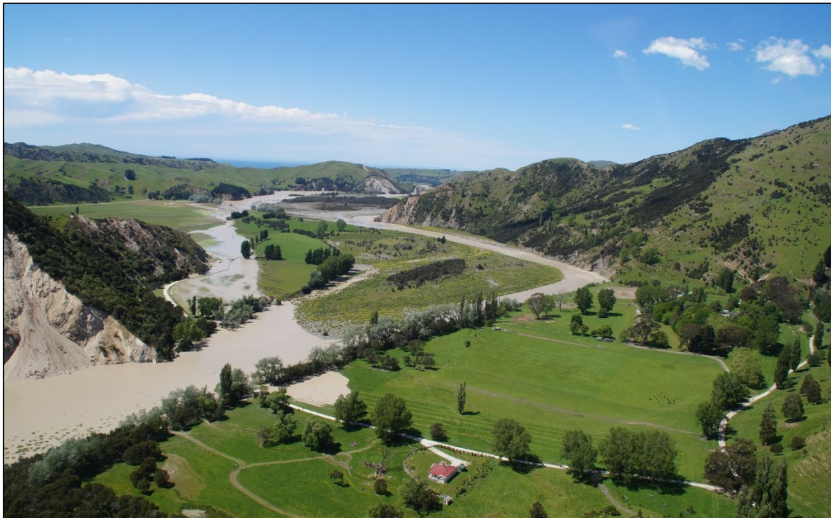
Figure 2-5: 15 November 2016 - Looking downstream along the Waiau Toa/Clarence River towards the Clarence Valley Road bridge site and Woodbank Station overflows
