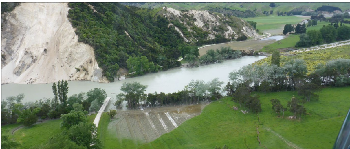
Figure 2-8: 25 November 2016 - Clarence Valley Road bridge site with Woodbank Station stopbank constructed post-2016 Kaikōura Earthquake Sequence
