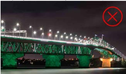
Auckland Harbour Bridge. Image www.aecilluminazone.com
