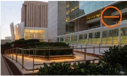
US Court House Annex, San Diego, California. Image source unknown.
