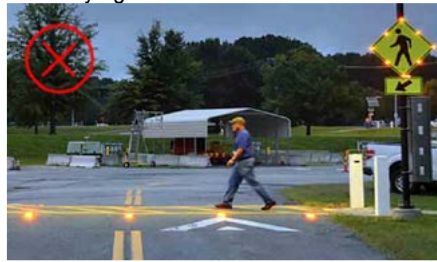
Flashing LED Pedestrian Crossing. Image Tapconet.com
