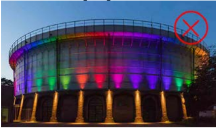
Westergasfabriek Amsterdam Netherlands Image CLS Lights .
