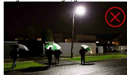
Failed LED retrofit Palmerston North, NZ. Image source unknown..
