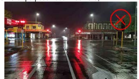
Failed LED retrofit Oamaru, NZ. Image Damien McNamara.
