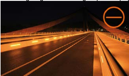
Amber LED lighting Pedret Bridge, Girona, Spain. Image Ignia Lighting .
