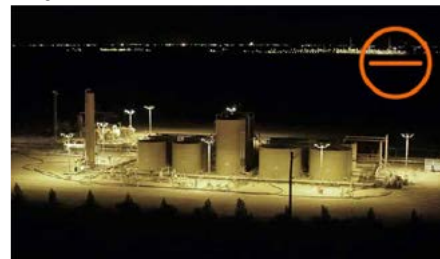
Apache/Altus Midstream Tank Battery, Reeves County, Texas.
