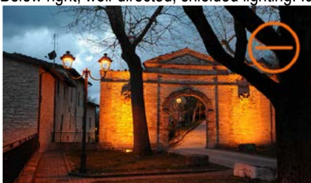
Sassoferrato, Italy. Image Neri Lighting .
