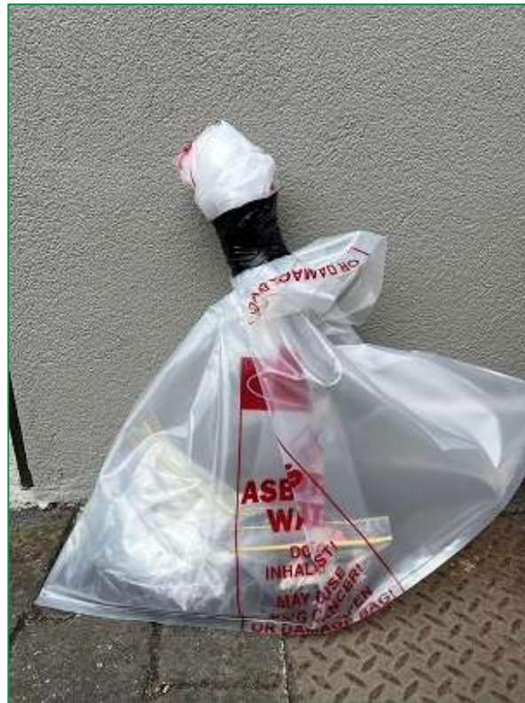
Figure 3. ACM prepared for disposal
