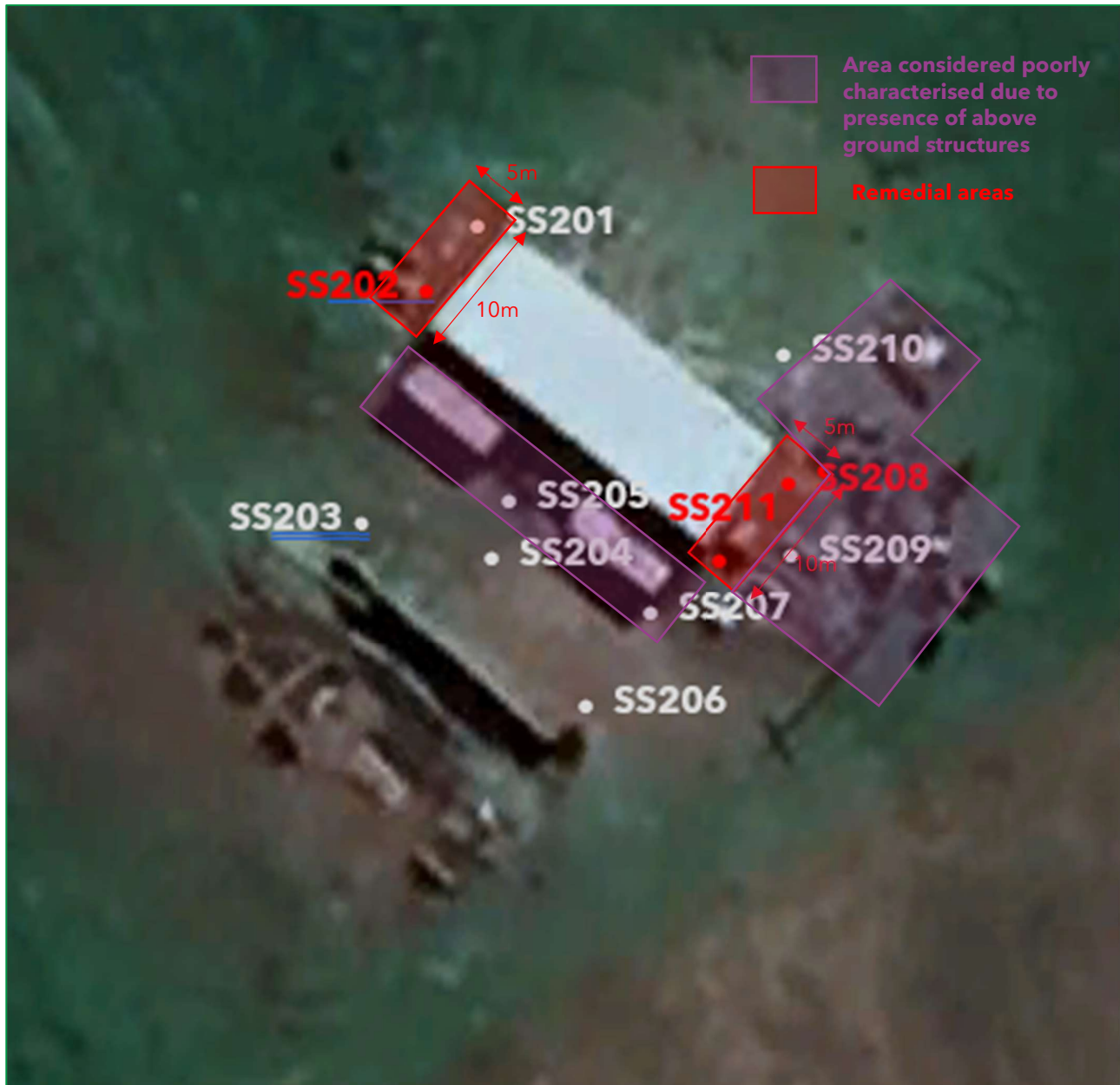
Figure 9. Area with Health Significant Asbestos Present to a Depth of Approximately 0.15m
