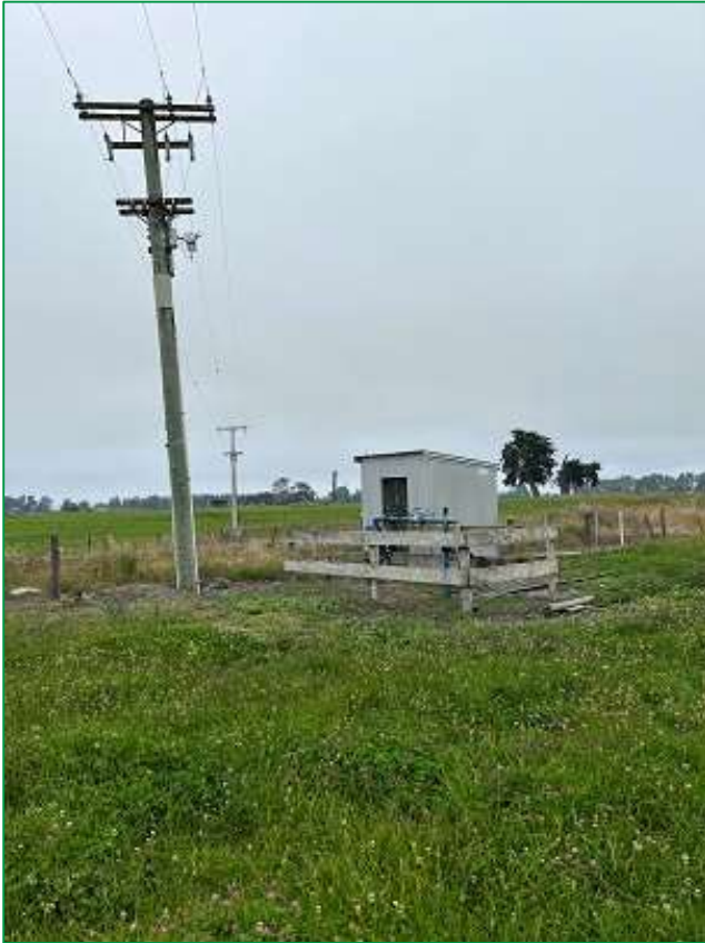
Photo 3 Well O31/0323 and pump house
