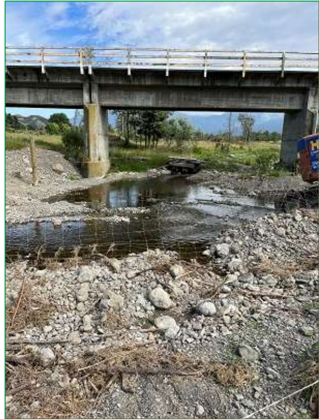
Photo 2 Stoney Creek at the railway bridge
