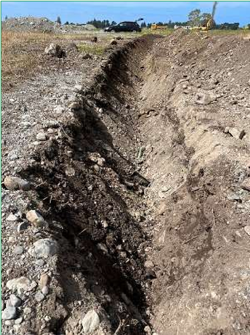
Figure 8. Trench in 'Piggery/Offal Pit' Area
