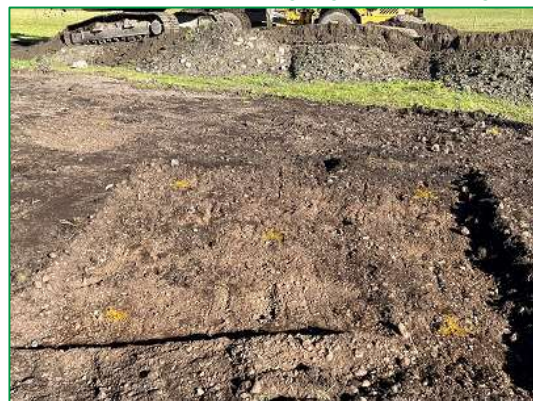
Figure 3. Images from the Remedial Work (Including Additional Excavation of Areas Returning High XRF Readings)
