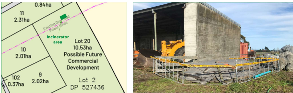
Figure 2. Temporary Stockpiling of Asbestos Contaminated Soil in the Incinerator Area
