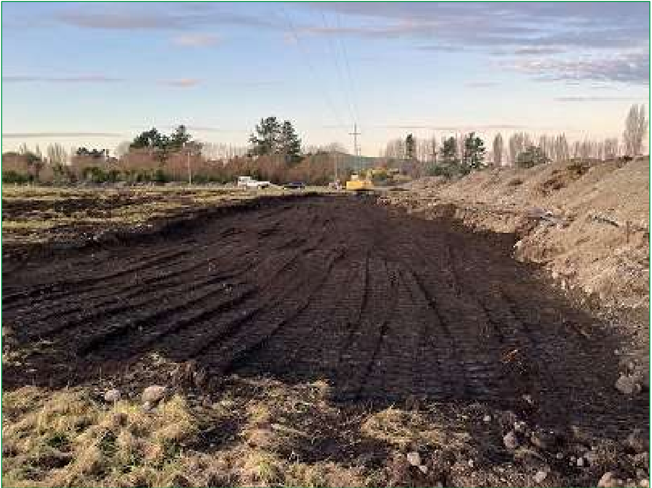
Figure 5. Containment Cell View to the East
