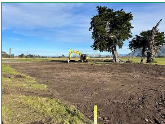
Figure 3. Images from the Remedial Work (Including Additional Excavation of Areas Returning High XRF Readings)
