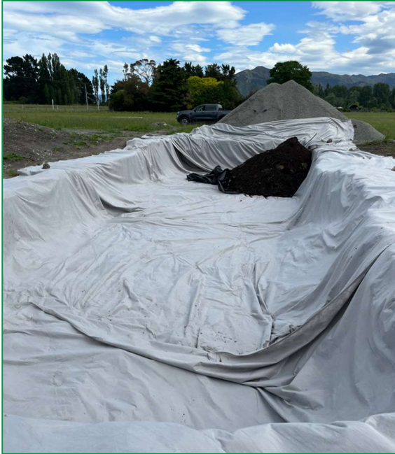
Figure 6. Containment Cell (red). Photographs show: 1. Geotextile layer on top of waste, 2. Topsoil on top of geotextile, 3. Gravel aggregate on top of topsoil. Basemaps from Baseline Group and Canterbury Maps
