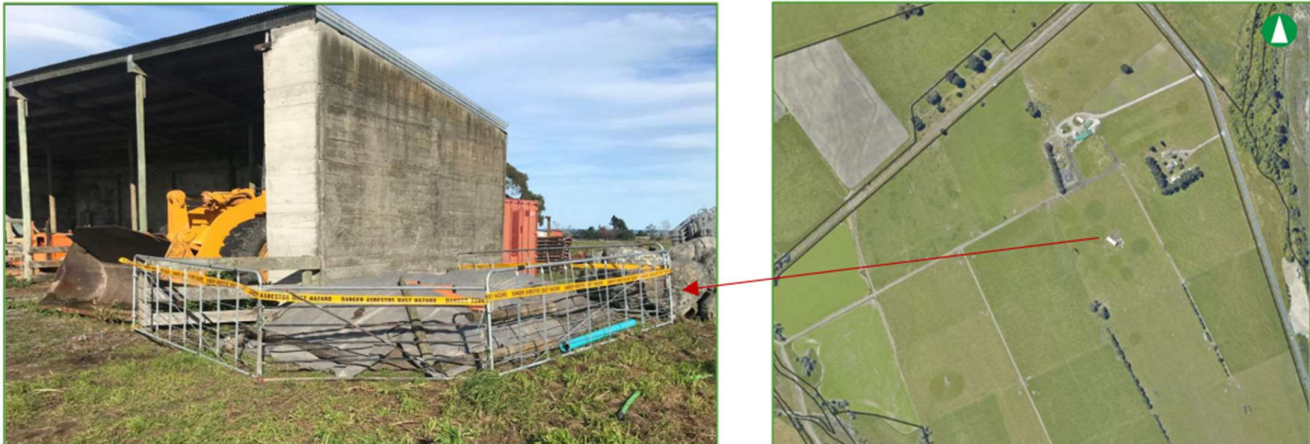
Figure 4. Temporary Stockpile of Asbestos Contaminated Soil at Northern End of Haybarn. Stockpile originating from the Historical Piggery Area in Lot 14. Basemap from Canterbury Maps
