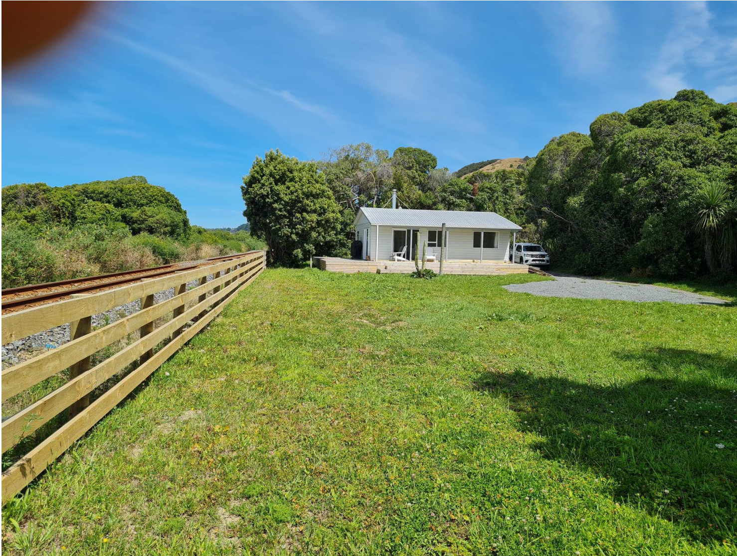
Existing Dwelling on Lot 2 from Lot ½ boundary looking south Proposed Subdivision of Pt Lot 1 DP 1033 – Kaikoura Trustee Company Ltd – 1516 State Highway No.1 - Mangamaunu, Kaikoura
