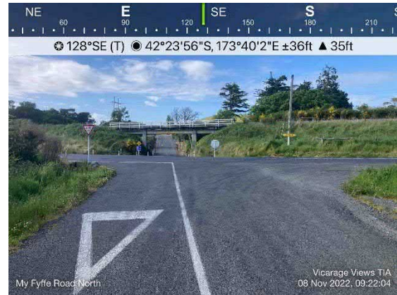
Figure 7: Ludstone Road/Mt Fyffe Road intersection (north)
