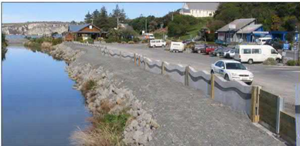
Figure 2-8: Lyell Creek flood protection wall
