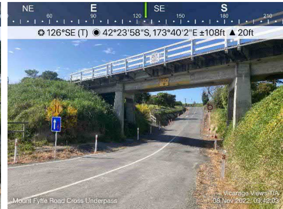
Figure 4: Mt Fyffe Road north of the railway overbridge
