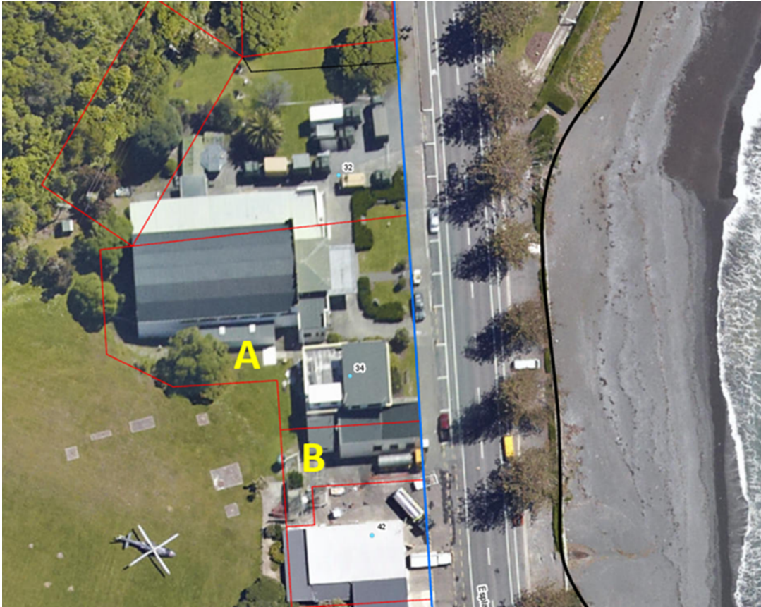
Figure 1: General Location – Old Council Offices at 34 Esplanade
