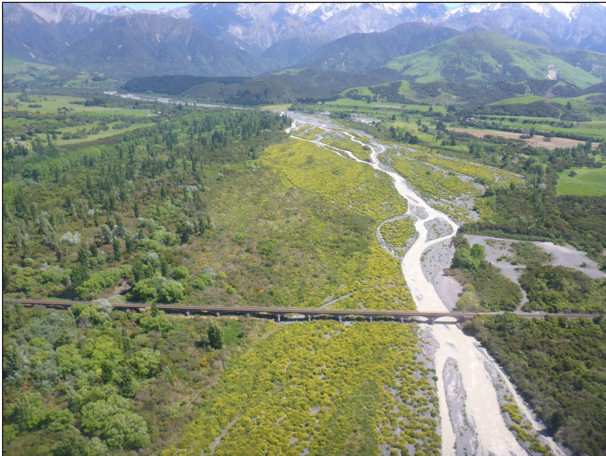
15 November 2016 – Looking upstream along the Hāpuku River towards the railway bridge
