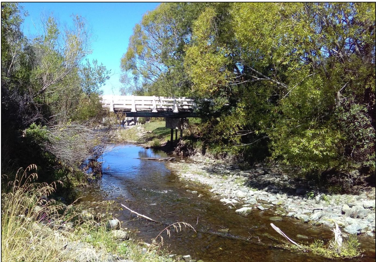
Figure 3-4: Ote Makura Stream looking downstream towards the campground road bridge
