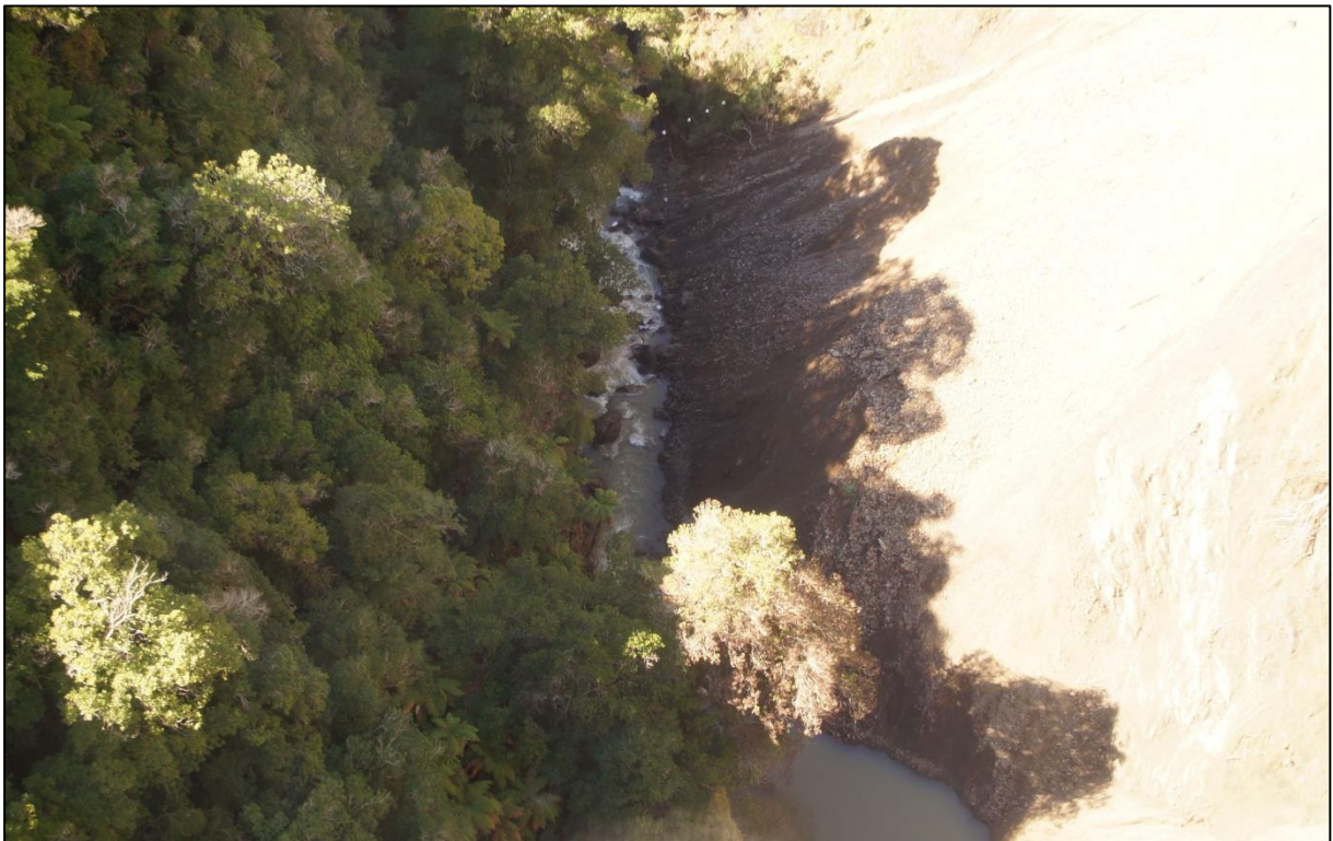
Figure 2-4: Ote Makura landslide dam on 7 April 2017 – looking downstream, from the lake area, at the channel cut through the landslide
