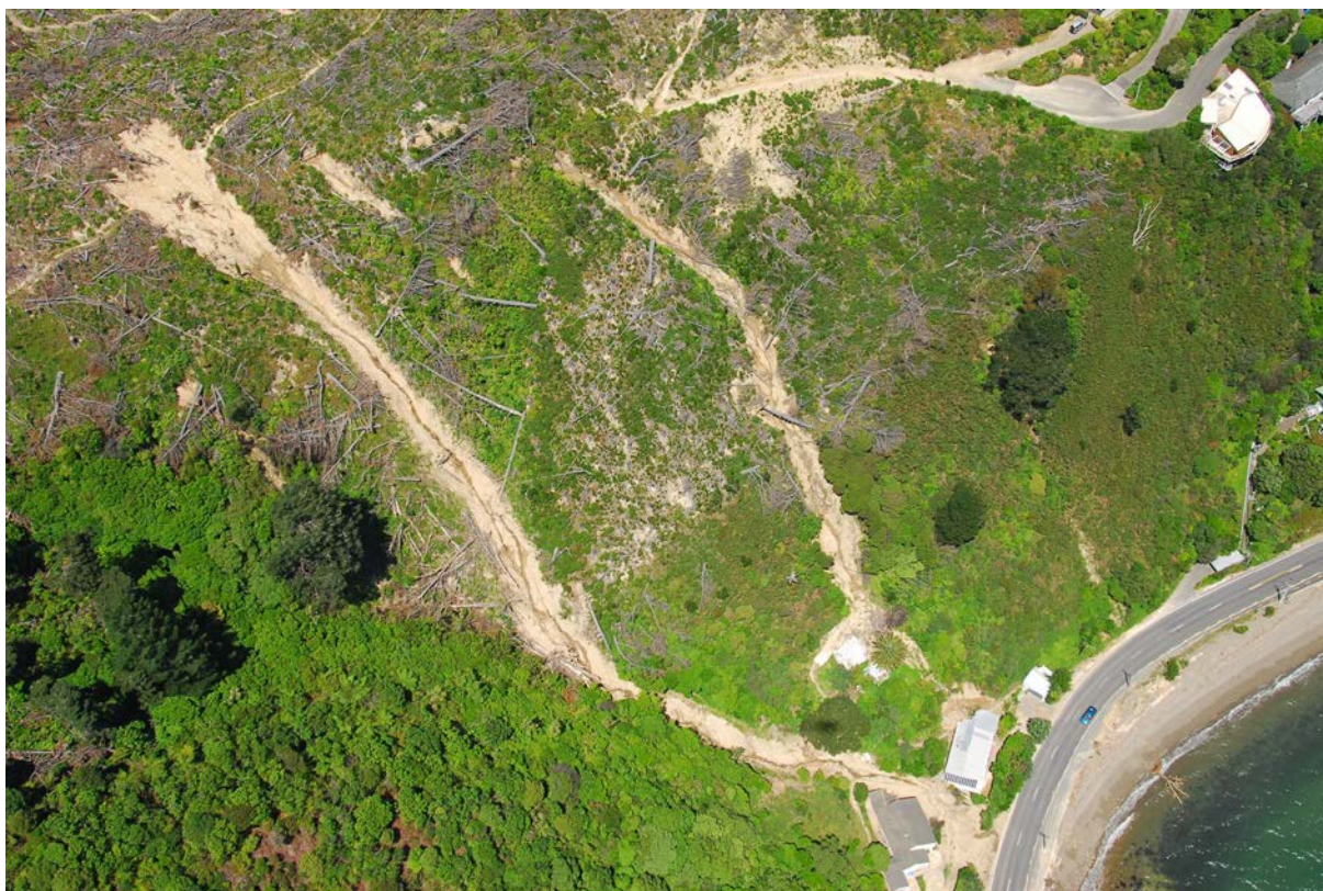
Figure 1.4 Debris flows triggered by rain in Eastbourne, Wellington, in November 2006. The source areas of the debris flows are in the left of the photograph. The debris travelled down slope several hundreds of meters where it impacted the dwellings shown in the right of the photograph. Photograph by G. Hancox, GNS Science.
