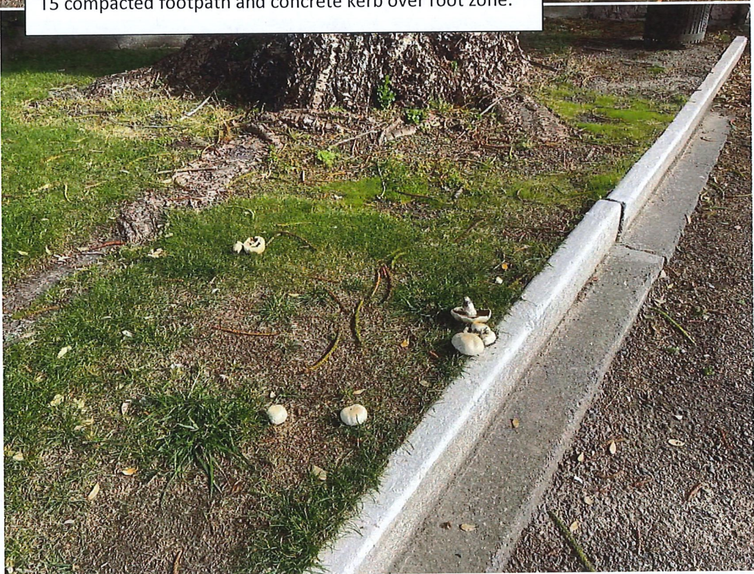
T5 compacted footpath and concrete kerb over root zone.
